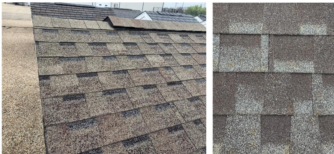
**Figure 3: Asphalt Shingles In-Service at Bloomington, IL Aging Farm (State Farm TRAIL)**
